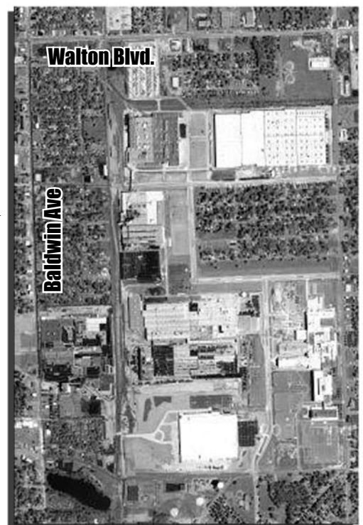
Current view of the plant 2009
